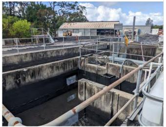
Plate 4.13 Oil water separator capturing runoff from the oil storage facilities, diesel tank storage, workshop / maintenance areas and wash bay
