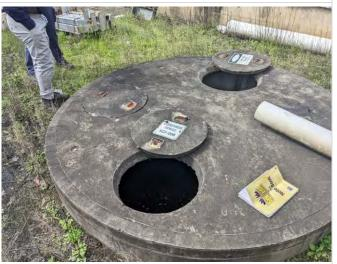
Plate 4.16 Oily water separator for compressors
